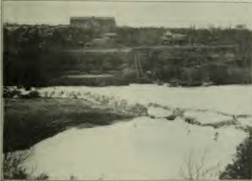
FIG. 3. ONTARIO POWER COMPANY'S POWER HOUSE ALMOST BURIED UNDER THE ICE.
